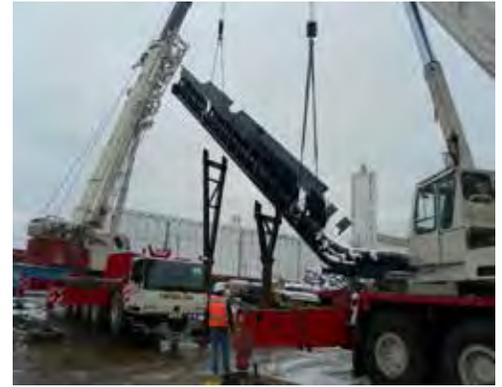
The Fenner Dunlop ECS team used two cranes to set the metal apron conveyor in one assembled piece that weighs 105,000 lbs. The tail of the conveyor had to fit into a concrete bunker with only ½” of clearance on each side.
